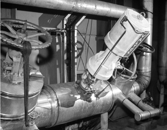
A 4-in Mark One with side-mounted handwheel operates a boiler feedwater system at a pulp plant.
